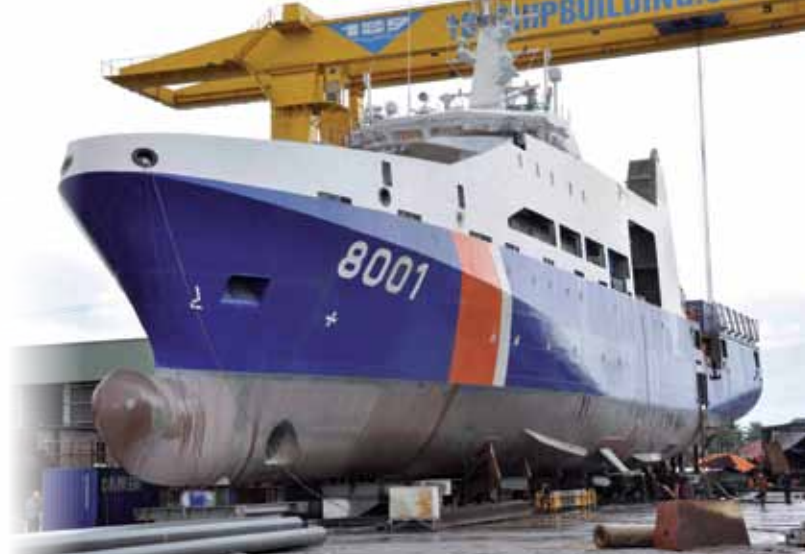
DAMEN OPV'S OPV 2400 under construction at regional yard under Transfer-of-Technology Program.
